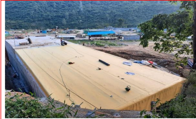
Waterproofing services of rooftop at Arunachal Pradesh
