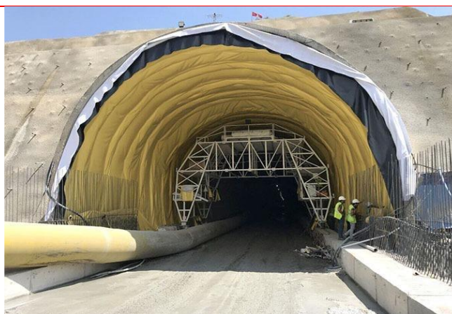
Waterproofing services of tunnel at Maharashtra
