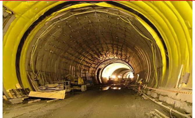
Waterproofing services of tunnel at Odisha
