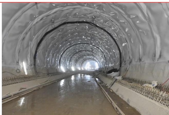
Waterproofing services of tunnel at Himachal Pradesh
