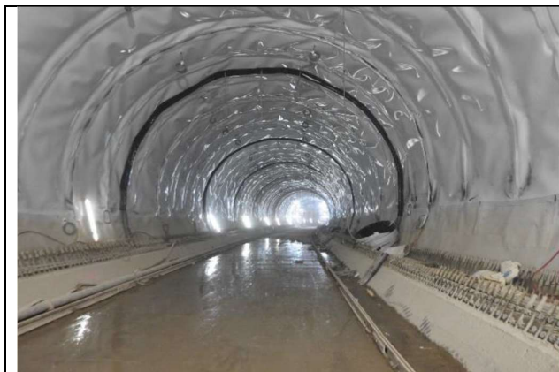
Waterproofing services at of tunnel at Himachal Pradesh
