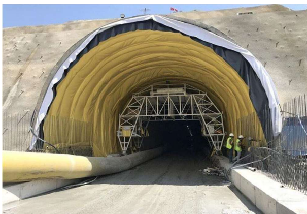
Waterproofing services of tunnel at Maharashtra
